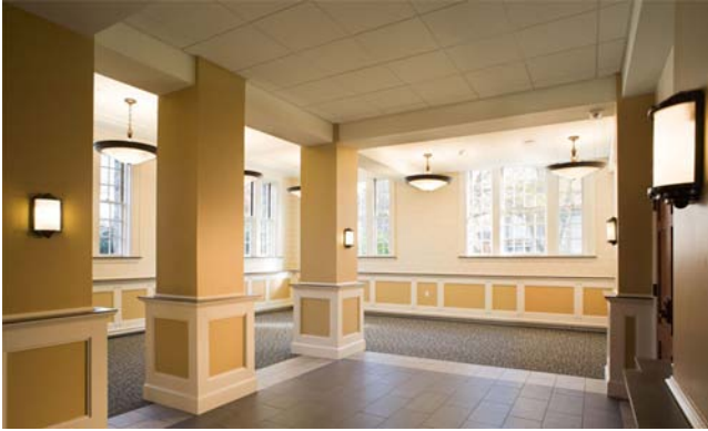
FIGURE 14. Theatre Sconces, MDF millwork, Corian sills.
