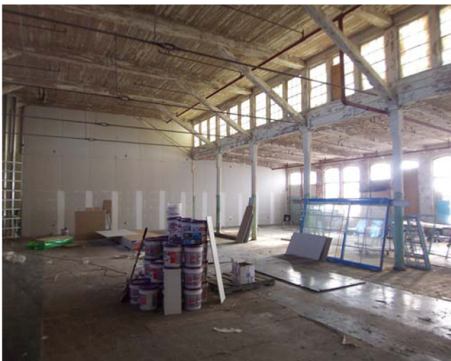
FIGURE 11. Mill building monitor before.
